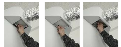
Hot air can be deflected into the room for heating in winter months
